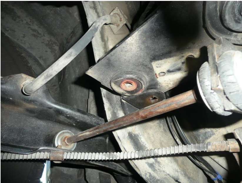
Figure 3 Left side crossmember moved rearward, left side.
