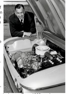
was convoluted induction with a choke fitted to the central air cleaner. From 1962, each carburetor had its own air cleaner.
