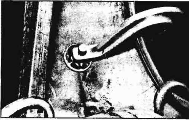
Fig. 3-40—Using Hot Patch Clamp
