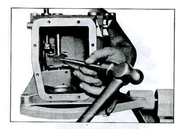
Fig. 7A-18—Installing First and Reverse Shift Fork
