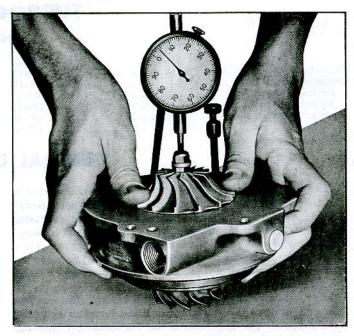
Fig. 37-Gauging Turbine Shaft End Play
