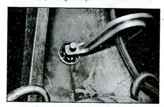
Fig. 10-Using Hot Patch Clamp
