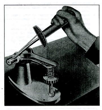
Fig. 83-Checking Valve Spring Tension
